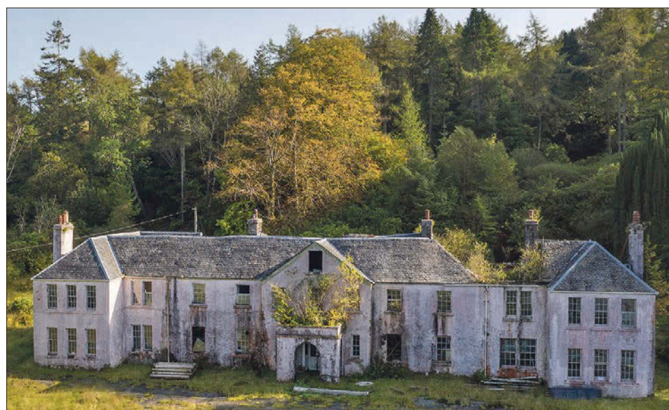
Pennyghael House, once owned by Genesis, but now needing full restoration or demolition.
