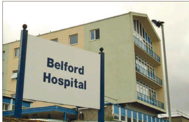
The Belford Hospital in Fort William.
