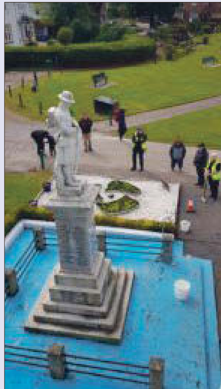
The start of the clean up, with assistance from The Highland Council Mobile lift vehicle.
