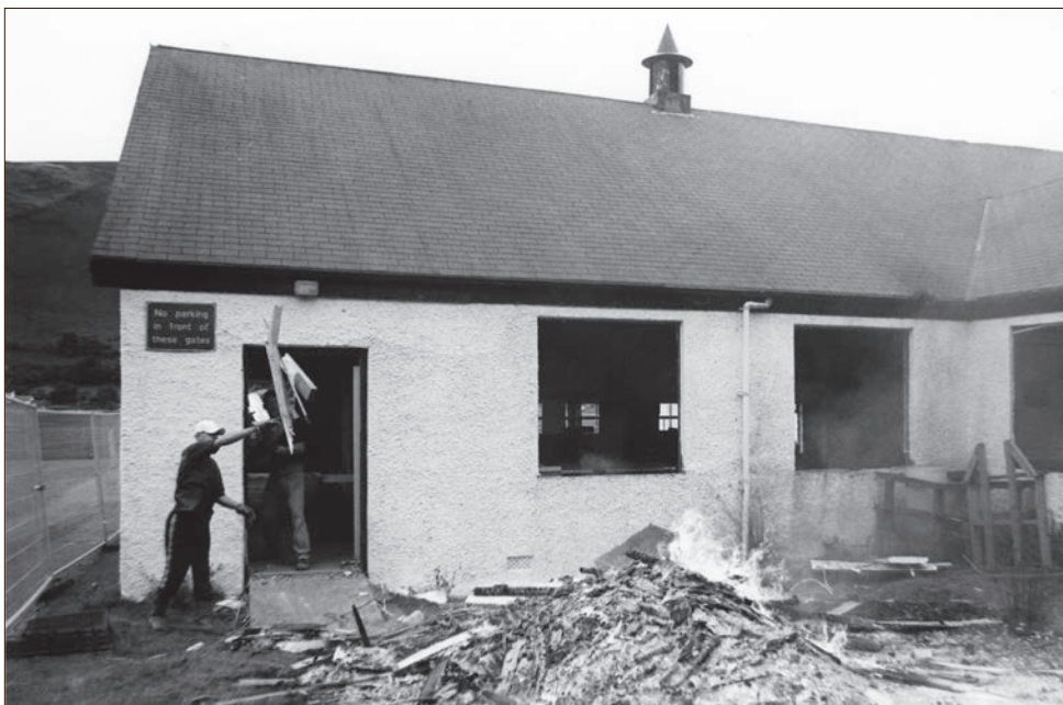
The old Lochranza hall will soon be no more as demolishers have been taking it to bits before bulldozing the walls. 01_B37years05
