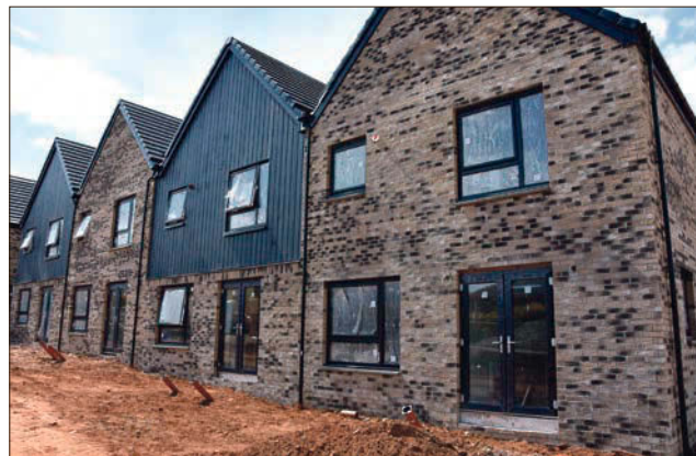
The new council houses nearing completion in Brodick.
