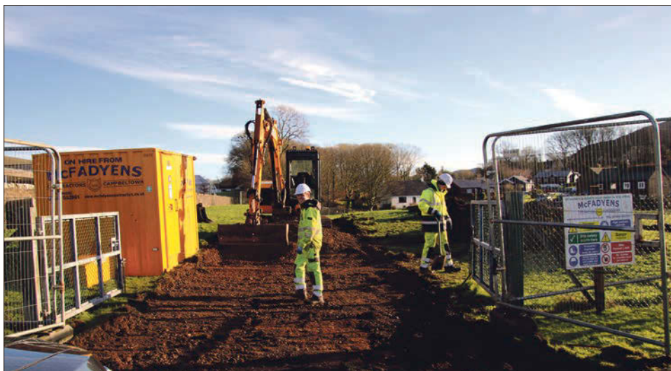
McFadyen's Contractors began construction of the Robert Black Memorial Helipad on Monday. Photograph: Kenny Craig.
