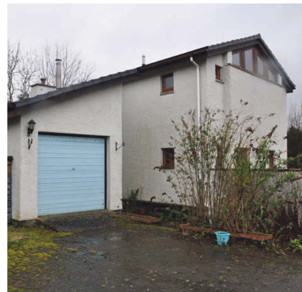
The Brodick Church manse which is to be demolished. 01_B08manse01
