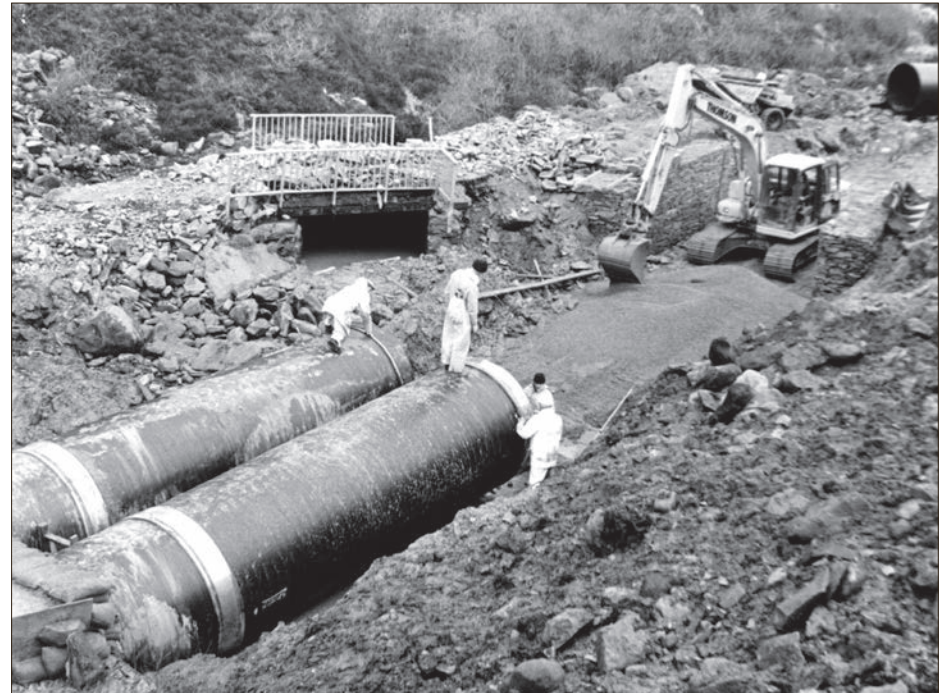
Major engineering works are ongoing at the Iron Bride on the Ross Road, which is closed to traffic at the moment. The burn itself has been re-routed and these enormous pipes are being placed in the original course of the burn. It seems likely that the route will have a slightly different route from previously, when it reopens. 01_B05twe05
