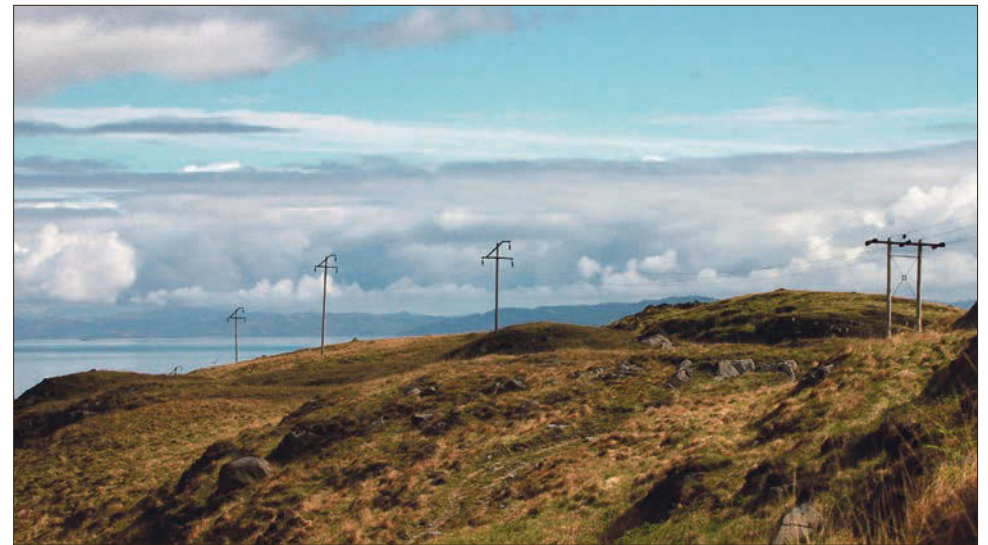
Jura's electricity network.
