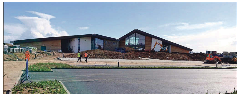
APRIL. With work on the new Lagg distillery nearing completion, the first batch of spirit already began last month with cask number one being filled this month.
