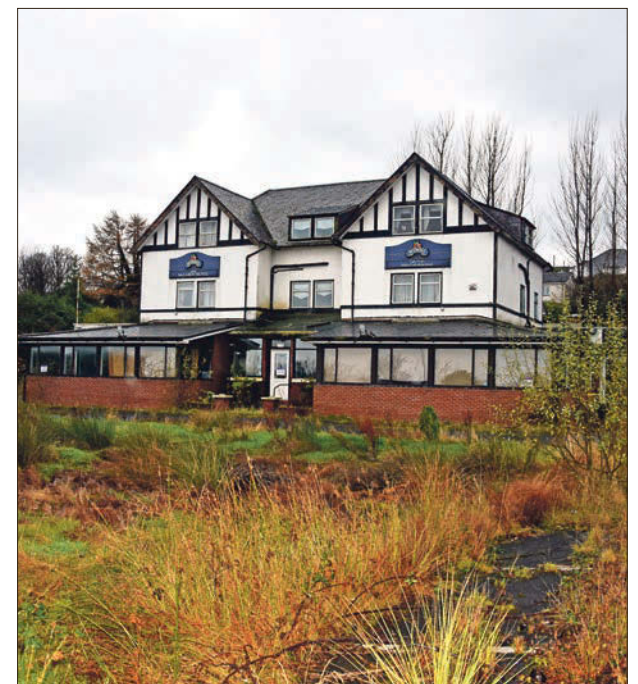
The McLaren Hotel lies dilapidated in its overgrown grounds this week. 01_B48mclaren01
