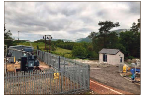
Work will be carried out at Taynuilt.
