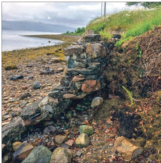
A section of damaged sea wall in need of attention.
