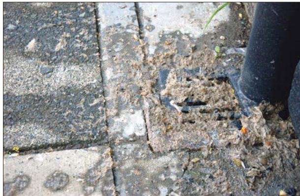
The increased capacity should help prevent scenes like this, pictured in Tarbert during June 2018. 06_a27TarbertSewage02
