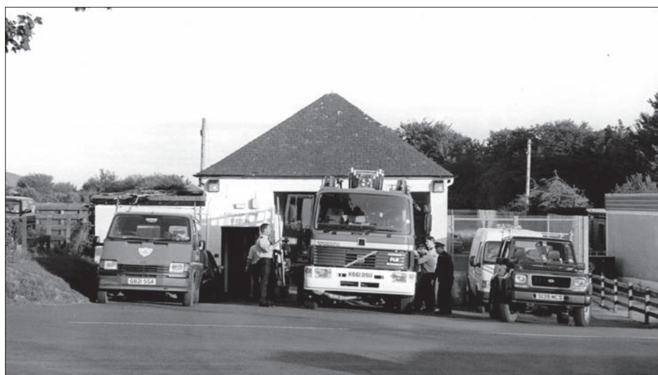
The old Lamlash fire station which had been in use since 1948. 01_B37twe02
