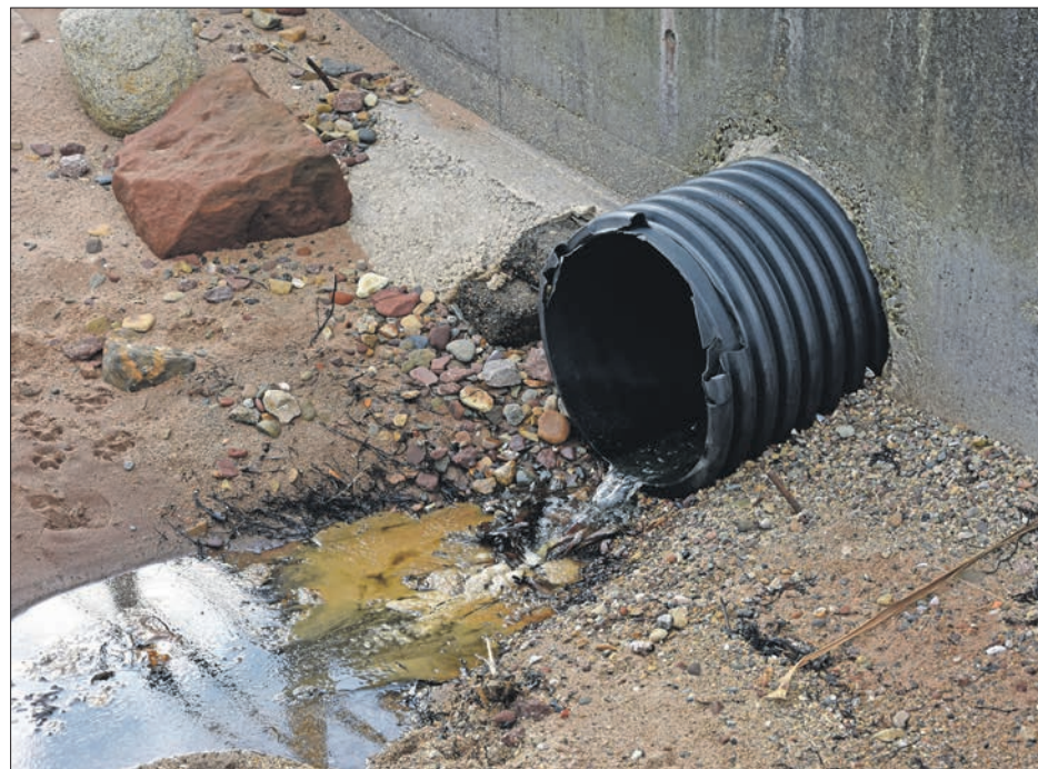
Domestic heating oil is evident at the outlet pipe near the Brodick slipway. 01_B35spill01
