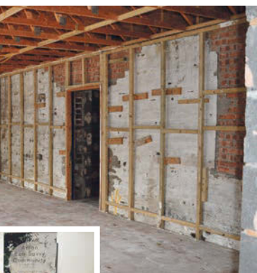
The inside of the cafe/restaurant has been stripped back 01_B30farm01; Charlotte Mann and Jude King in the new Eco Savvy office. 01_B30farm03
