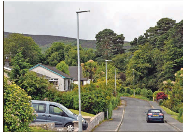
Street lights in a residential Brodick street which have been permanently lit for three months. 01_B25lights01
