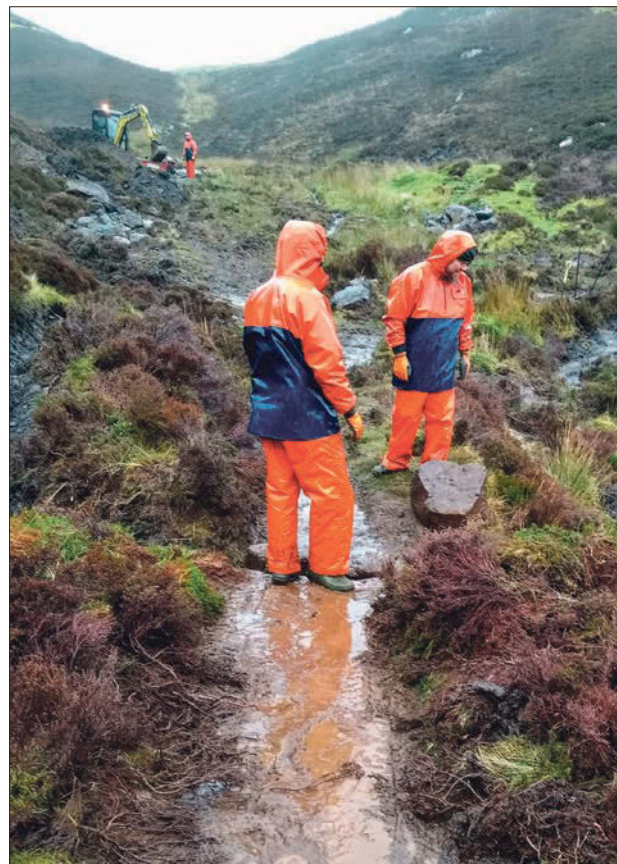
Arran Footpaths workers construct resilient water routes to prevent damage to the existing path.
