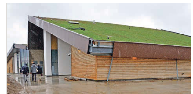
The natural living roof of the new distillery where work is still going on. 01_B18lagg25
