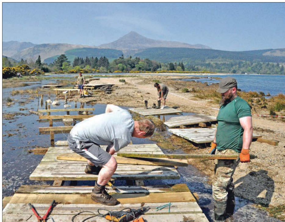
Liam Crawford and Josh Emmerson of Arran Footpaths and Forestry Ltd at work repairing the boardwalk. 01_B18boardwalk01
