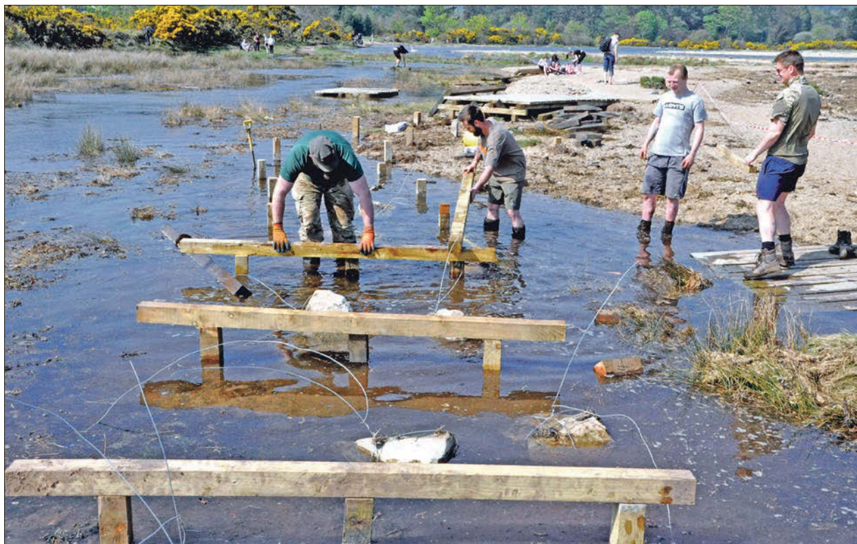
Deeper foundations have been dug to try to stop the boardwalk from being damaged again by storms.
