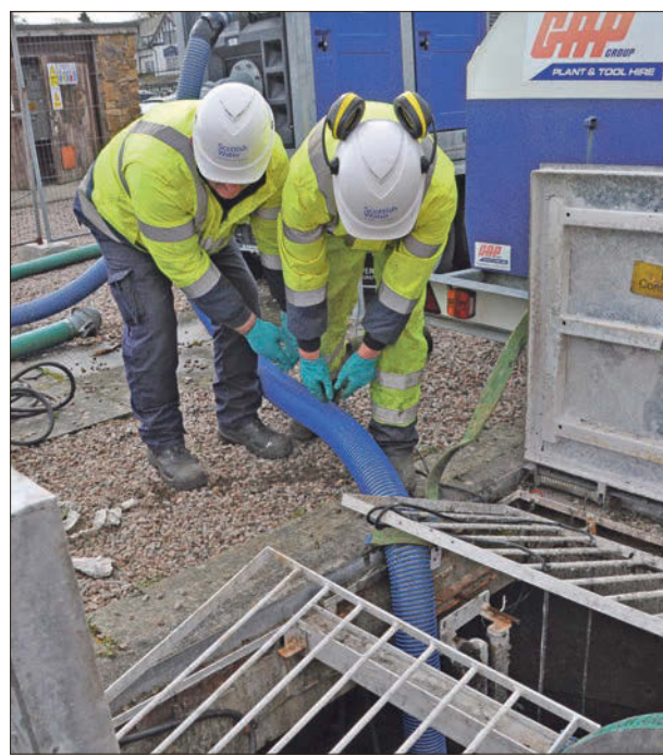
Scottish Water staff undertaking repair works in Brodick. 01_B16water02
