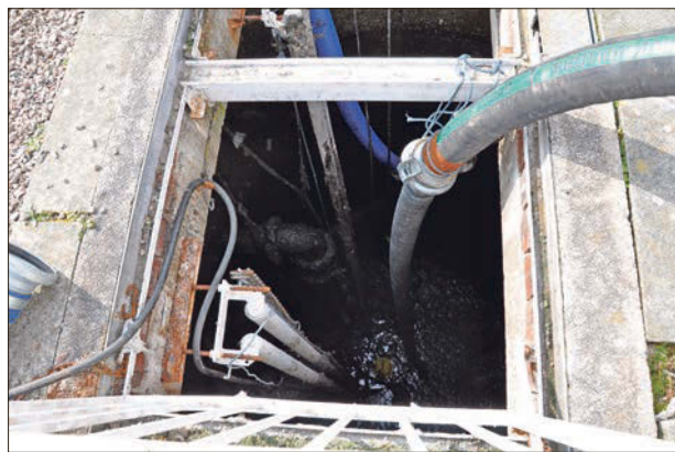
The yellow top of the electric pump can just be seen at the foot of the 20ft well. 01_B16water01
