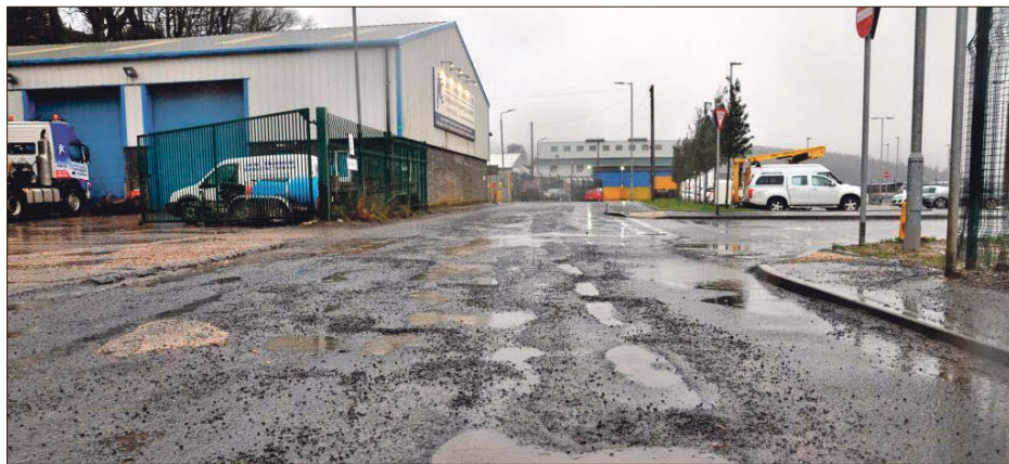
Potholes at the Brodick ferry terminal exit on Market Road which are due to be repaired.
