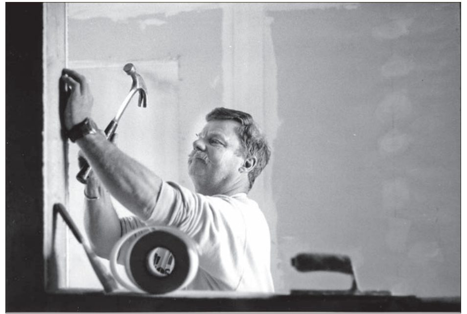
Keith I'anson of John Corbett Construction works on Corrie hall where refurbishment is nearing completion. 01_B16twe01
