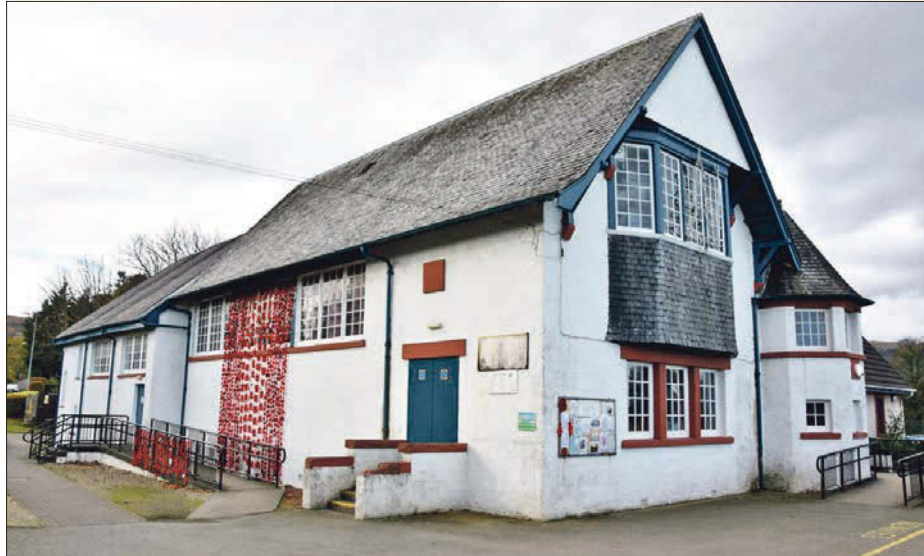
The Arran Library and Brodick Hall.
