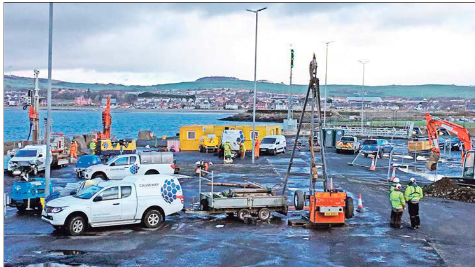
Preliminary works under way at Ardrossan harbour.
