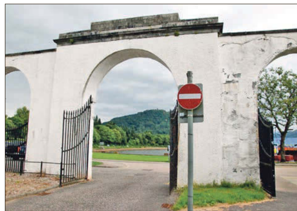
Above: the Avenue Screen was in need of some TLC before work began. 06_a31InvArch03
