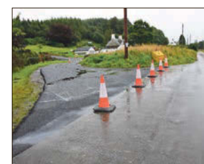
The new section of tar linking into the canal bank road. 51_a36Cairnbaandiversion02
