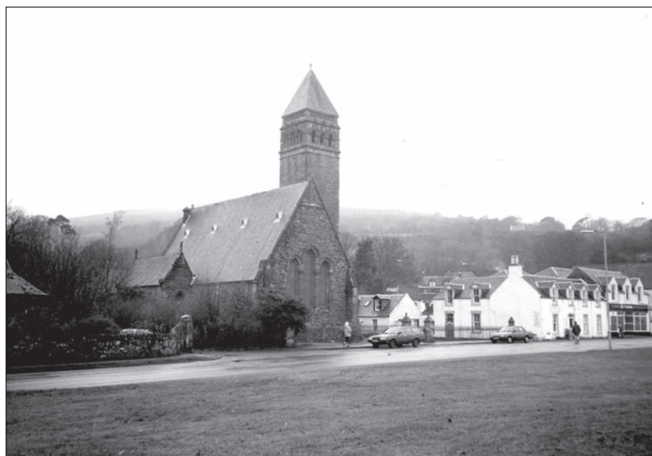
Lamlash Church members have been raising funds for over two years to repair their church which was originally built in 1886. The A listed building was a gift to the village by the Duke of Hamilton and features a nine bell carillon, one of only five in Scotland. B50twe05
