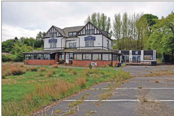
The site of the previous McLaren Hotel as it is at present.
