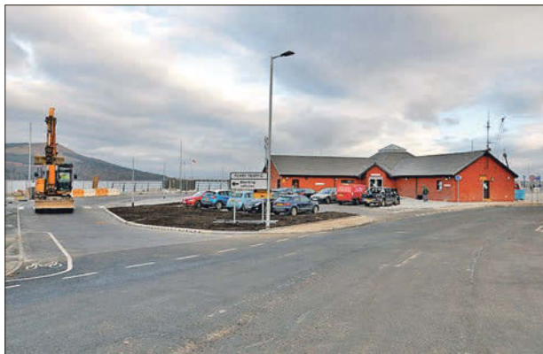
The new entrance for vehicle traffic leading to the marshalling area. 01_B49terminal01
