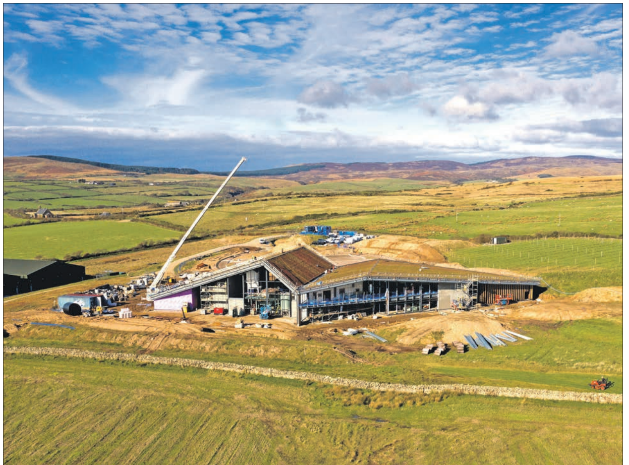
The Bauder roof of the distillery at Lagg is nearing completion as BHC Ltd crack on with the main contractor work.
