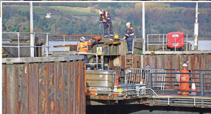
Services being removed from the linkspan. 01_B45pier03
