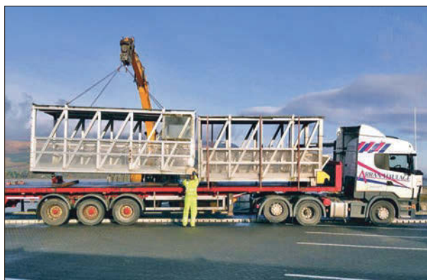
The former gangway is loaded on to a flatbed truck. Photo: Russell Duncan
