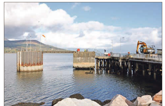
Part of the pier structure which will eventually be removed.
