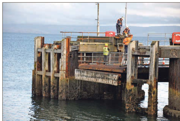
Dismantling work underway on the linkspan. 01_B45pier02
