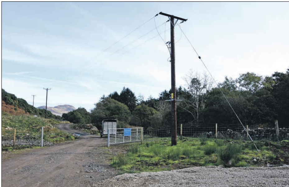
The powerlines carry the electricity to homes on Arran. 01_A44hydro14
