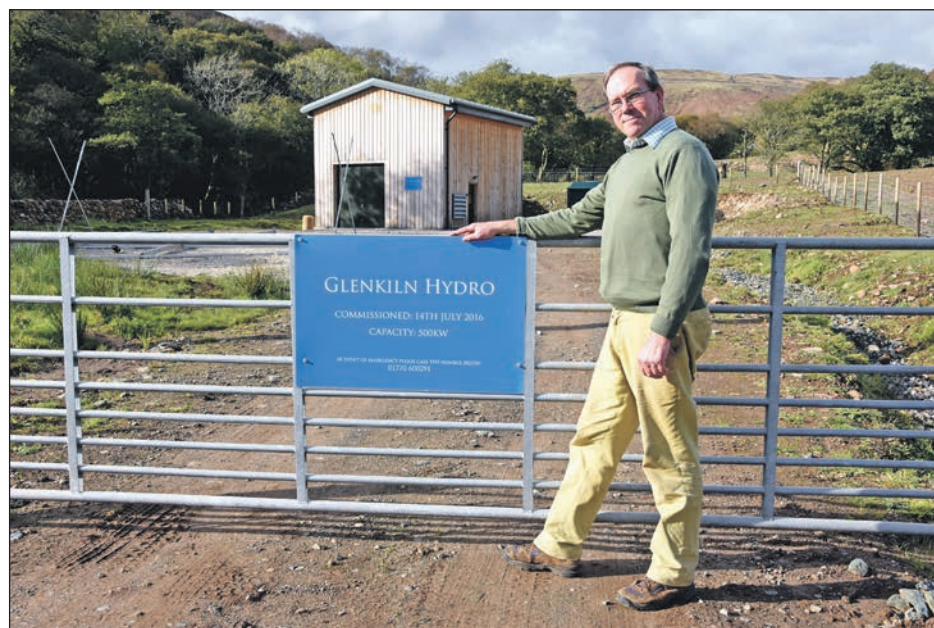
Kenneth with the Glenkiln Hydro sign showing the date of commission with the powerhouse in the background. 01_A44hydro01
