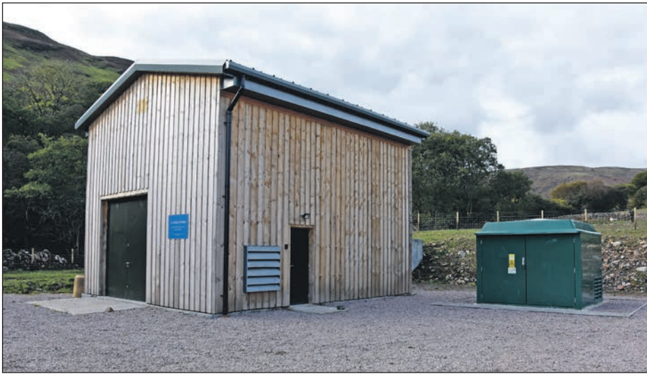
The powerhouse where the water is turned into electricity. 01_A44hydro13
