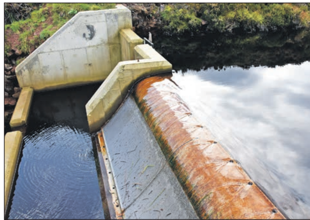
The water of the Benlister Burn flows over the inlet.
