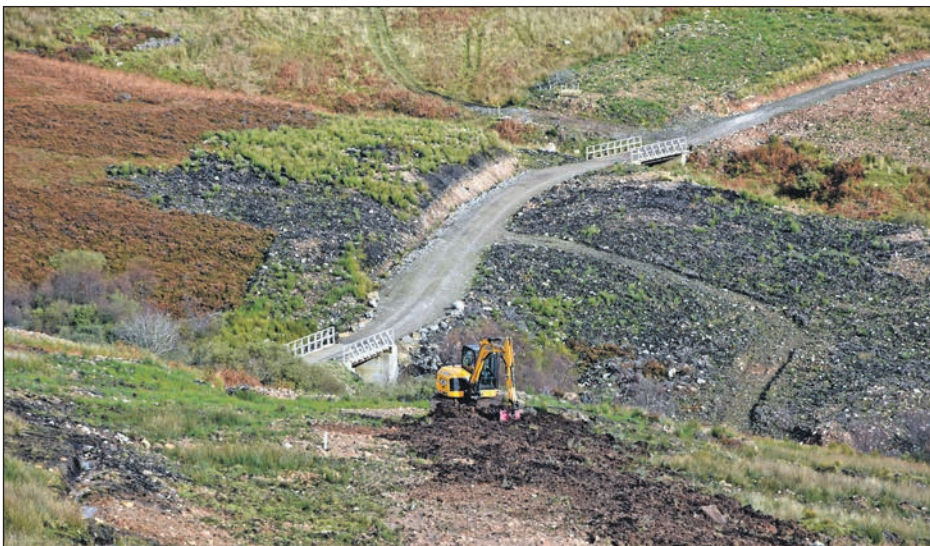
Two of the three bridges which had to be built to carry the road. 01_A44hydro11
