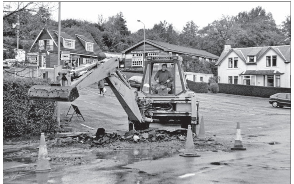
Clean-up operations take place in Whiting Bay where overflowing culverts raised the road and Tarmac which was submerged under the water. 01_B43twe01
