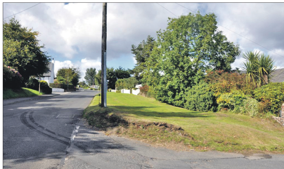
The site which been approved near Brableside for the new mast. 01_B37mast01
