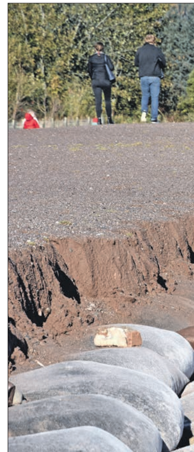
The geotextile bags lie exposed again as the beach crumbles into the sea.
