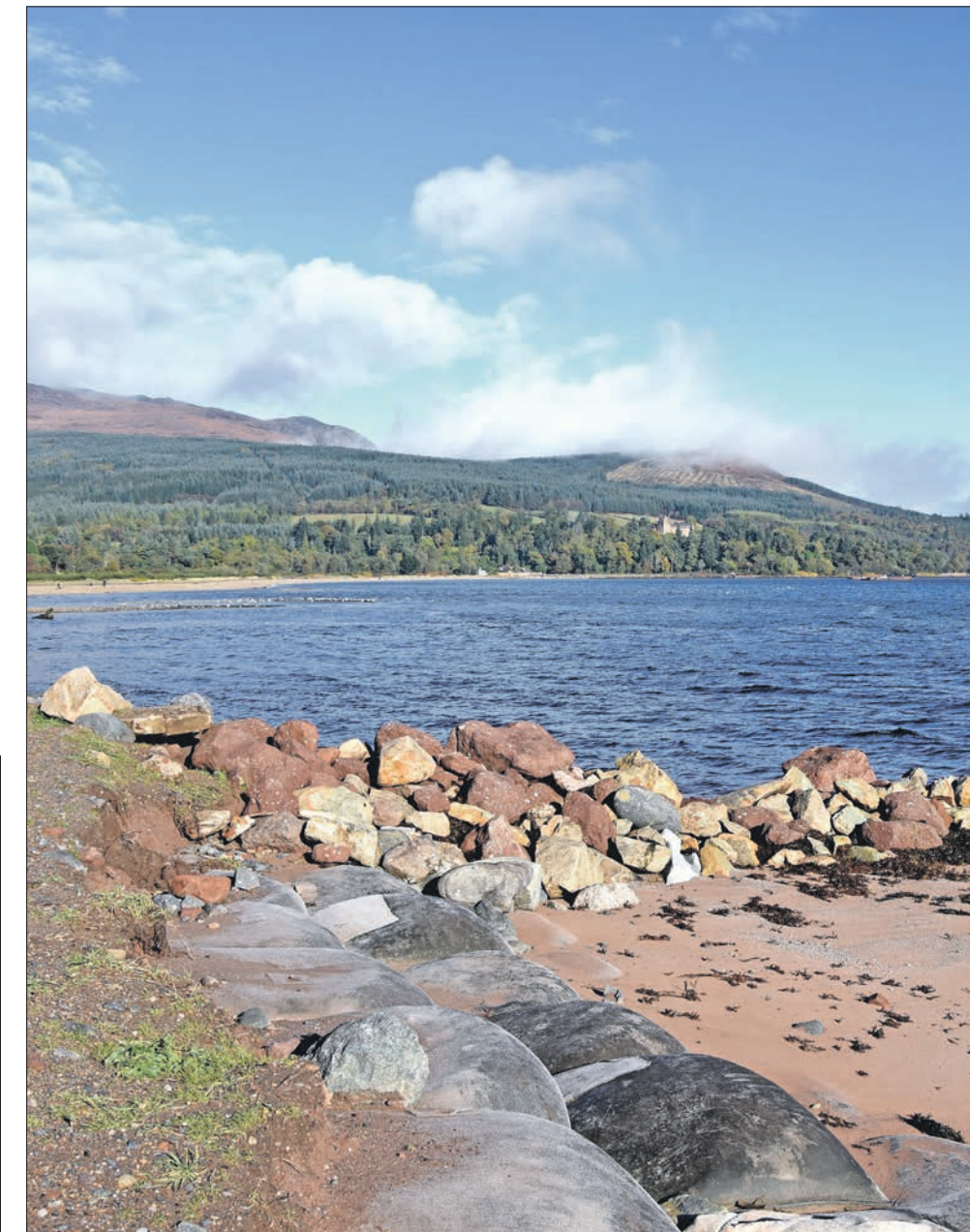
The initial groyne, although damaged, is doing some good. 01_A43beach03
