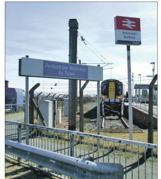
Ardrossan Harbour station.
