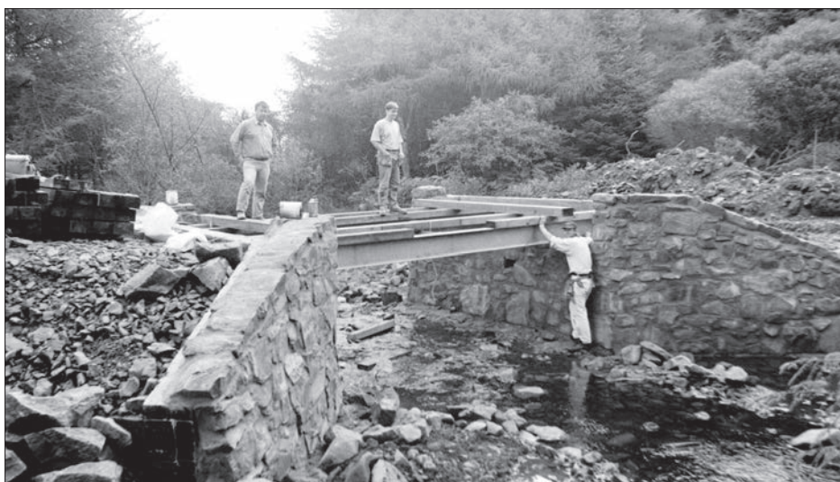
High above Glenashdale Falls, Graham Thomson, Neil Young and Paul Goody have been building a bridge. Making inroads into the forests of the southern half of the island, the new road and bridge will service heavy goods vehicles hauling timber. 01_B41twe05
