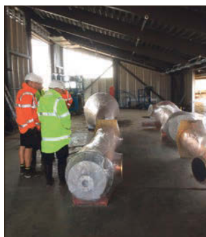
Master Distiller James MacTaggart and colleagues were on site to welcome the stills which will now be installed in preparation for a commissioning phase.
