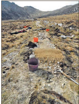
A section of path under repair. B34NTS02No
