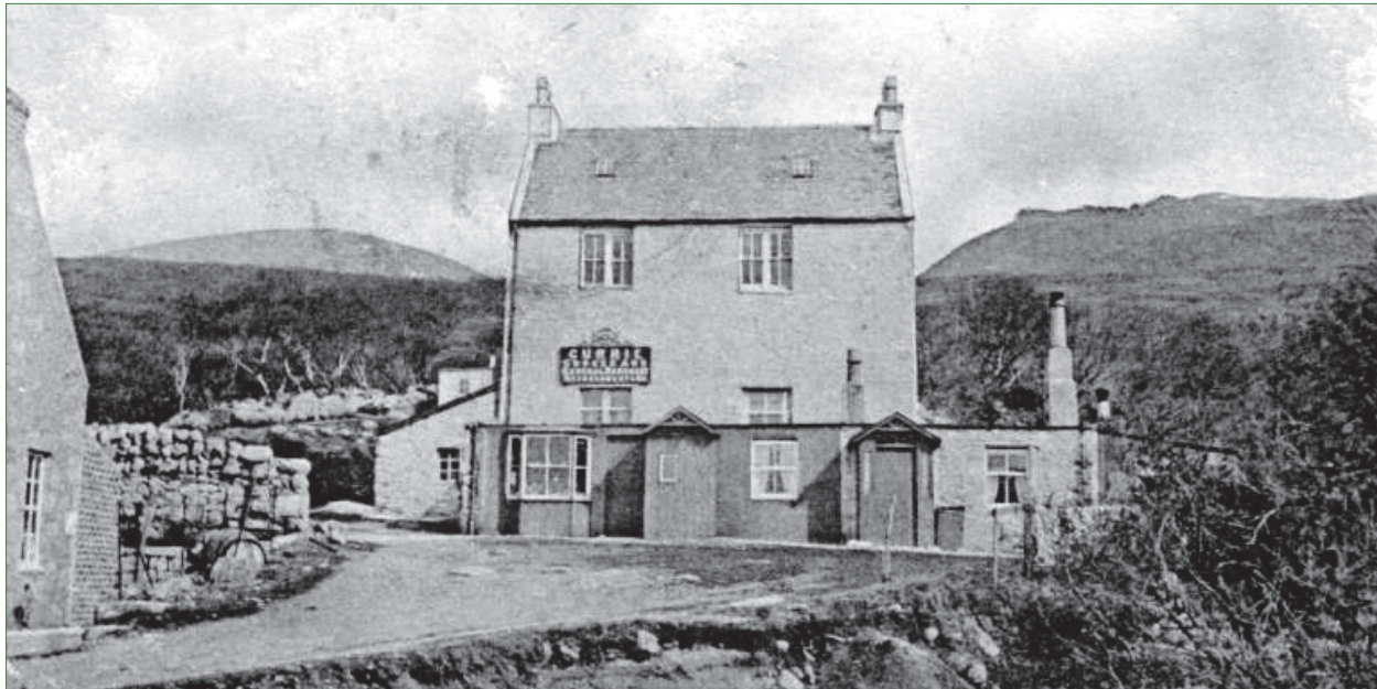
Eventually becoming Mill Curre's grocer's shop, Clark's old bobbin mill from which Pirnmill derived its name.
