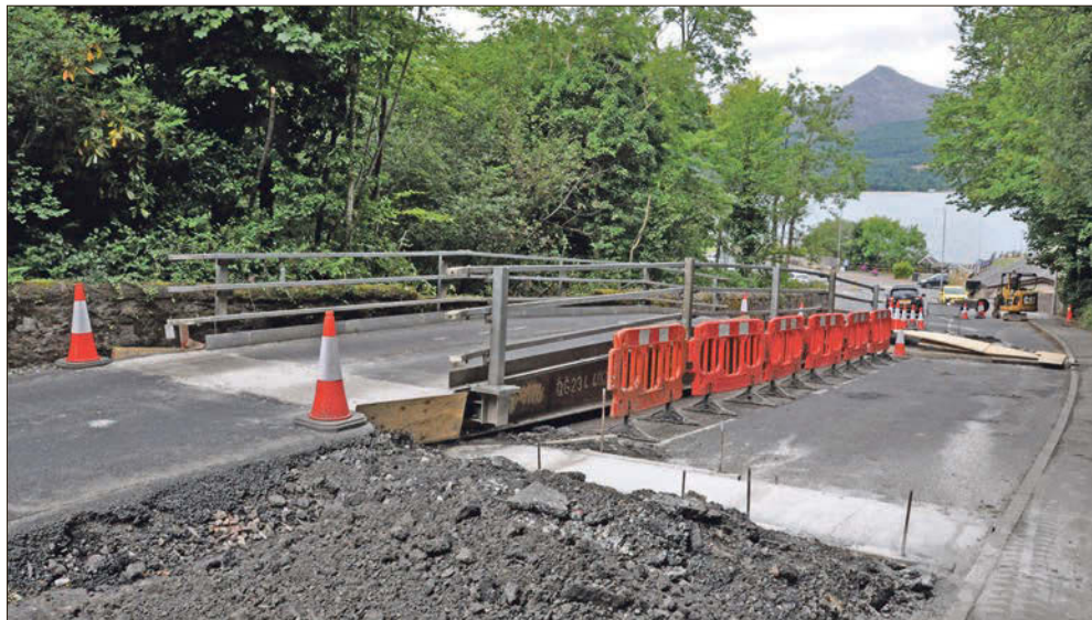
The first section of the new temporary bridge heading into Brodick. 01_B30bridge01
