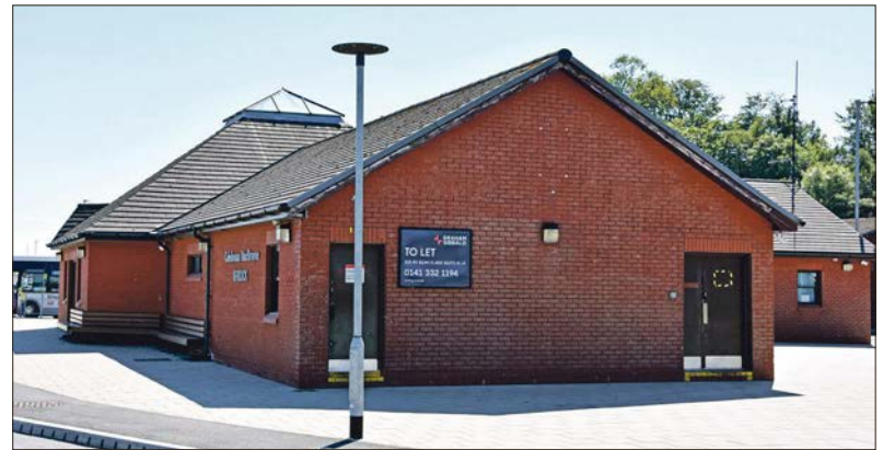
The Brodick ferry terminal which is available to let.
