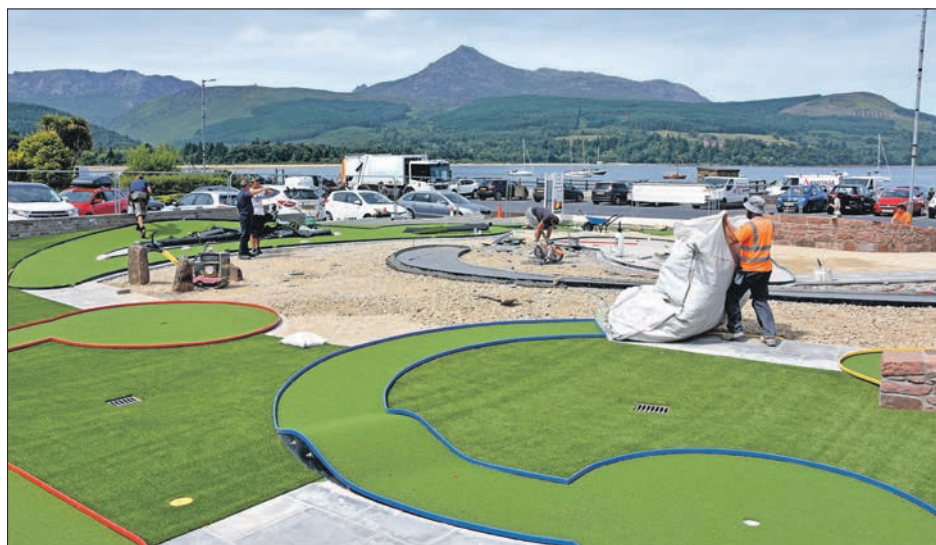
Workmen continue making good progress on the site with a few holes already nearing completion. 01_B26putt01
