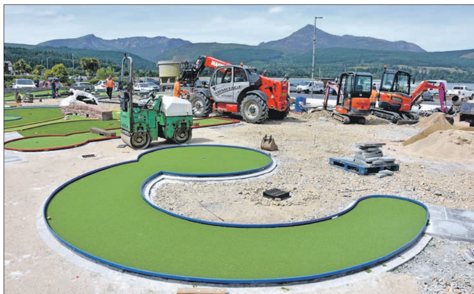
The last of the heavy machinery completes the remainder of the groundwork on the last holes. 01_B26putt02
