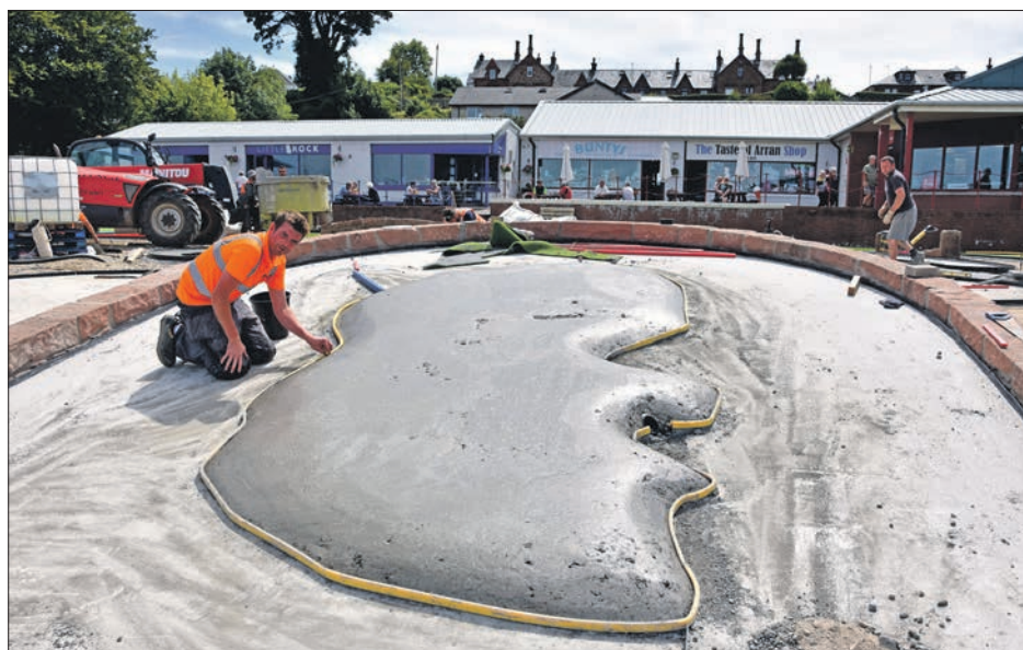
Workman Greg McCrae puts the finishing touches to the sculptured relief of the Arran shaped centrepiece. 01_B26putt03
