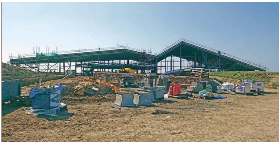
The iconic structure of the Lagg Distillery is rapidly taking shape.
