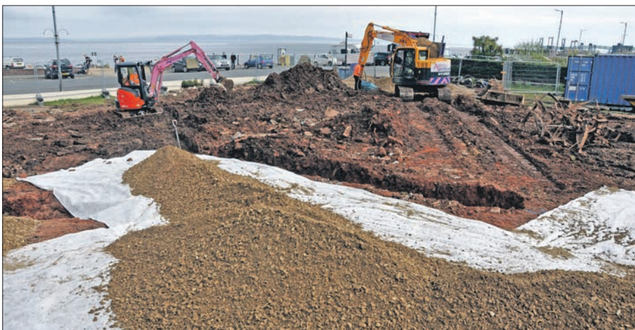
Mini diggers and landscaping machinery prepare the site earlier in the week. 01_B19mini02
