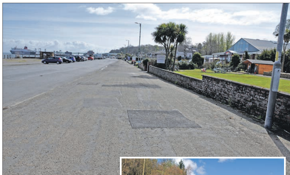
The aesthetics of the differing surfaces and badly maintained tarmac along Brodict is of concern to the trust. 01_B18civic03
