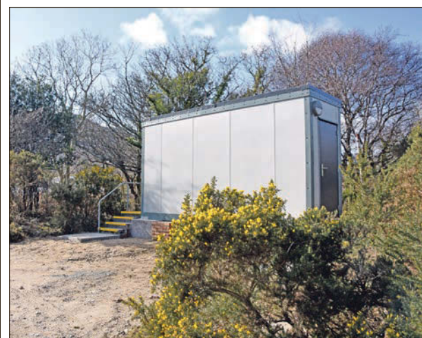
The new toilet block at Sannox. 01_B17toilet01
