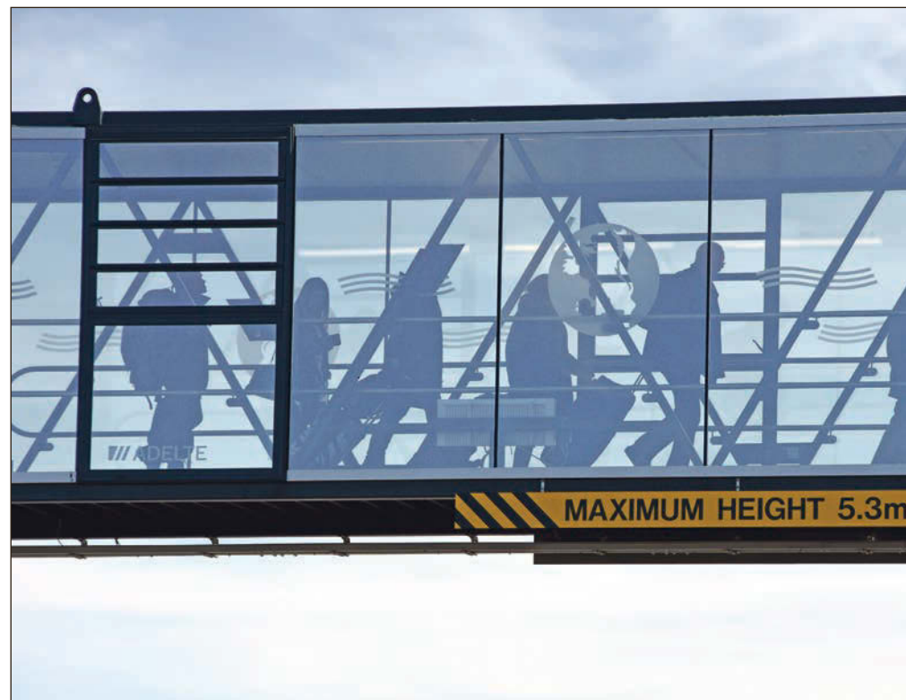
The passenger connecting 'tube' is just one of the areas of concern. 01_B17civic01
