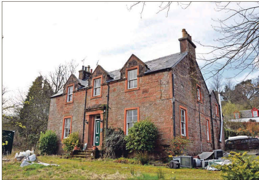
The Glencloy farmhouse is in a bad state of repair and is derelict. 01_B17glencloy02
