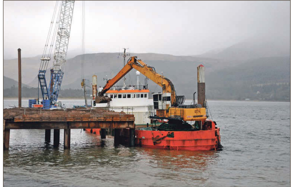
The MV Grete Fighter dredges the sand from the ferry terminal site. 01_B17sand07
