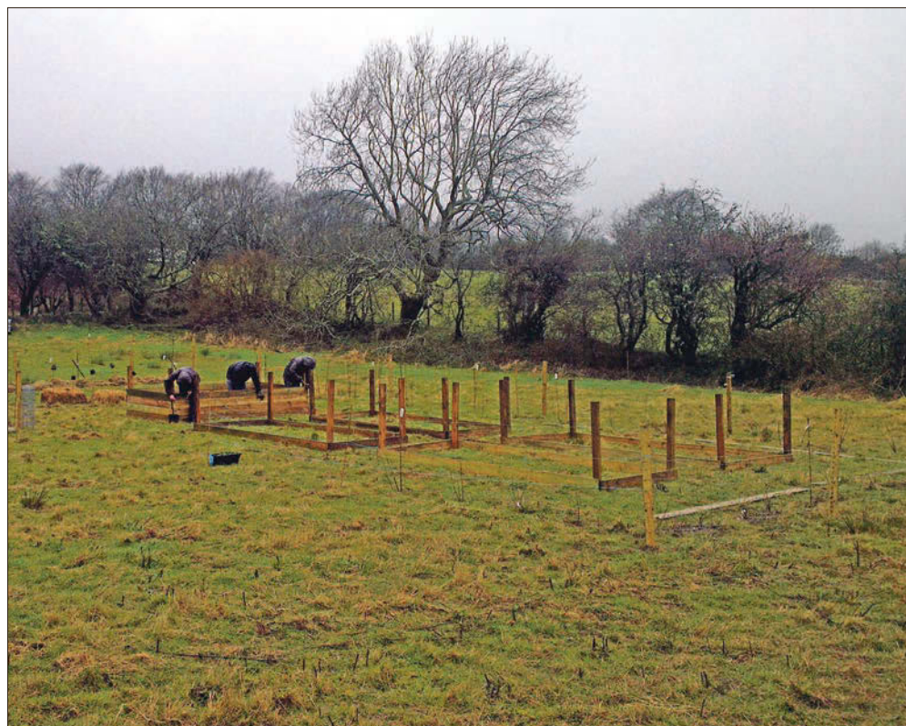
Volunteers can be seen working on building raised beds on the showcase allotment.
