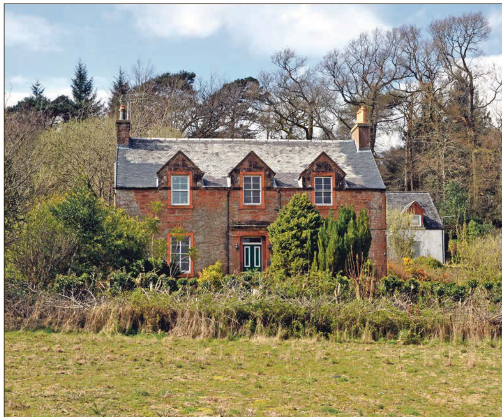
Glencloy farmhouse which might soon be demolished. 01_B17glencloy01
