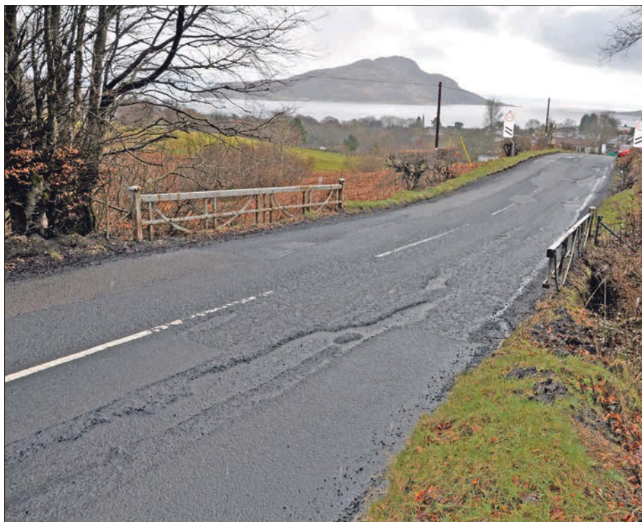
A badly rutted section of the road which is to be repaired in Lamlash. 01_B16roadworks01
