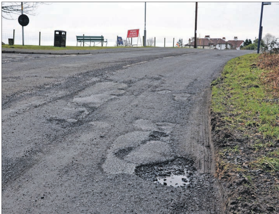
The road end at Sandbraes in Whiting Bay is pitted with potholes. 01_B08pothole01
