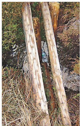
ABOVE and RIGHT: The Forestry Commission have had to spend a lot of money fixing tracks and bridges which bikes have damaged and broken.
