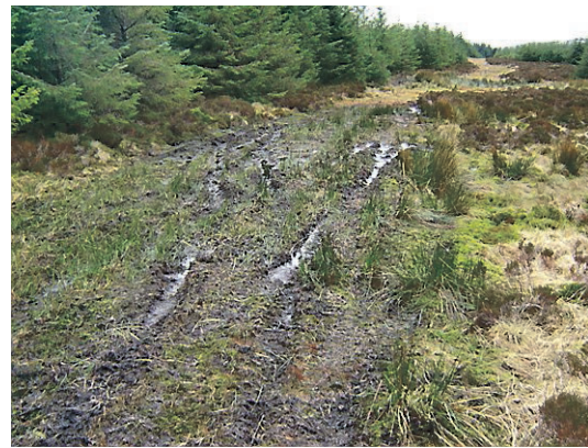
One of the tracks that has been severely damaged the tracks being damaged. We have a strict no vehicle policy in those tracks.
