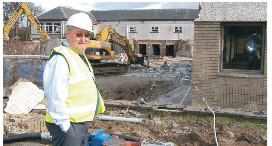
Contractor Iain Thomson on Wednesday, just before the start of the demolition of the old school main building. b12ian01
