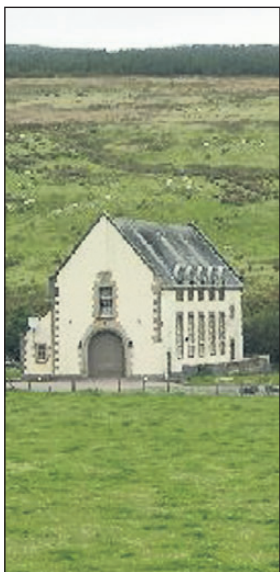
Glen Lussa power station near Peninver.
