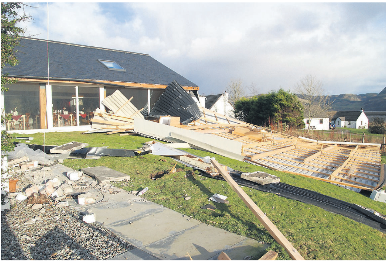
The Galley of Lorne Inn at Ardfert had its roof ripped off at the height of the storm. t03r004
