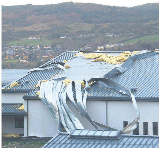
Large sections of Lochgilphead Joint Campus' roof were torn off by the storm. A02sch01
