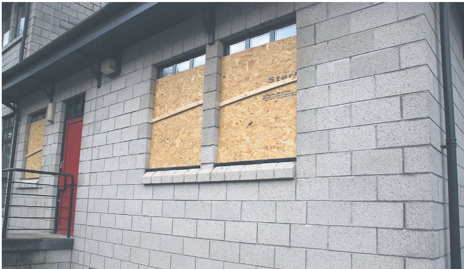
Windows boarded up on Manse Brae after vandals struck at New Year. A02win01
