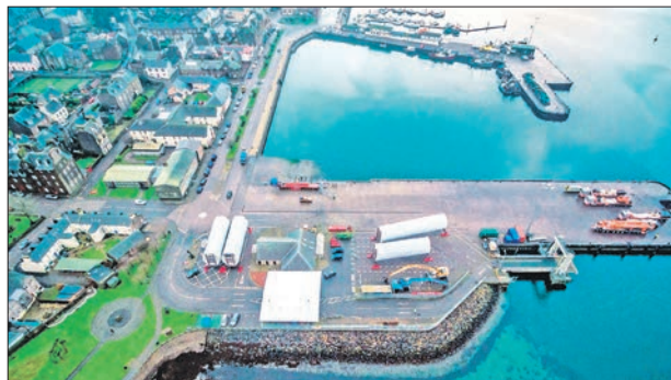
The tower sections from the air on Campbeltown's new quay. Photographed by licensed drone pilot Raymond Hosie.
